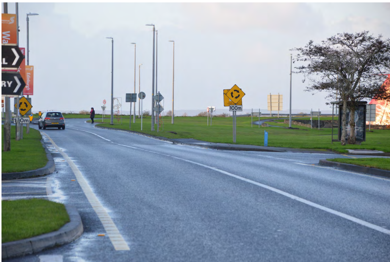
Plate 5-11: Existing Bus Stop
